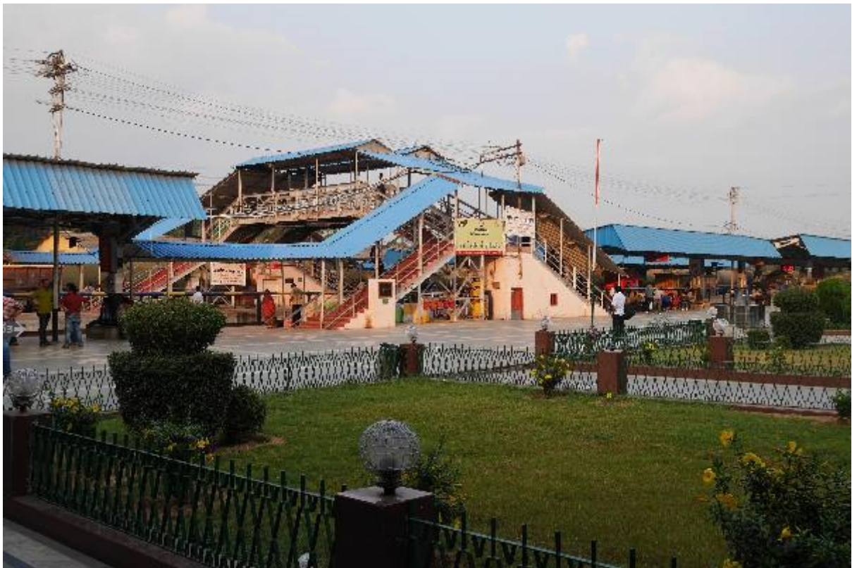
Sambalbur Junction station
